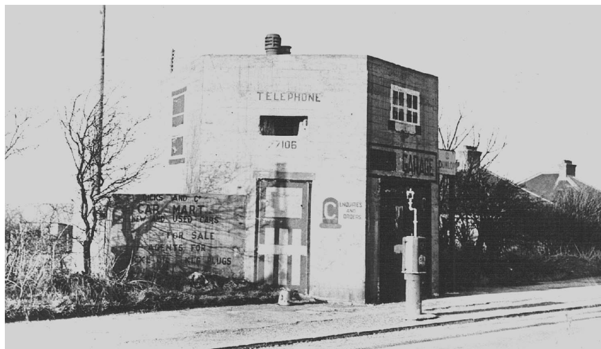
Two-story pillbox disguised as Garage at Capel-le-Ferne, Folkestone. Note petrol pump, advisements, chimney pots.
